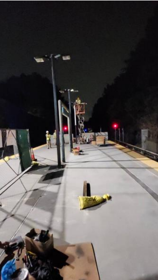
Platform- Concrete/ Lighting
