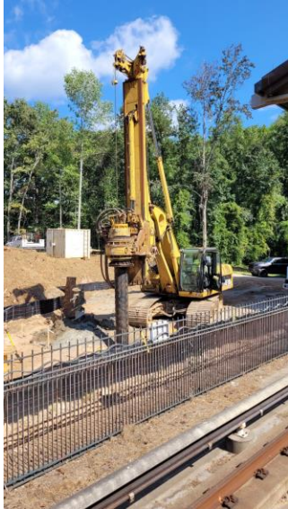
North/ South Property- Foundations for Bridge
